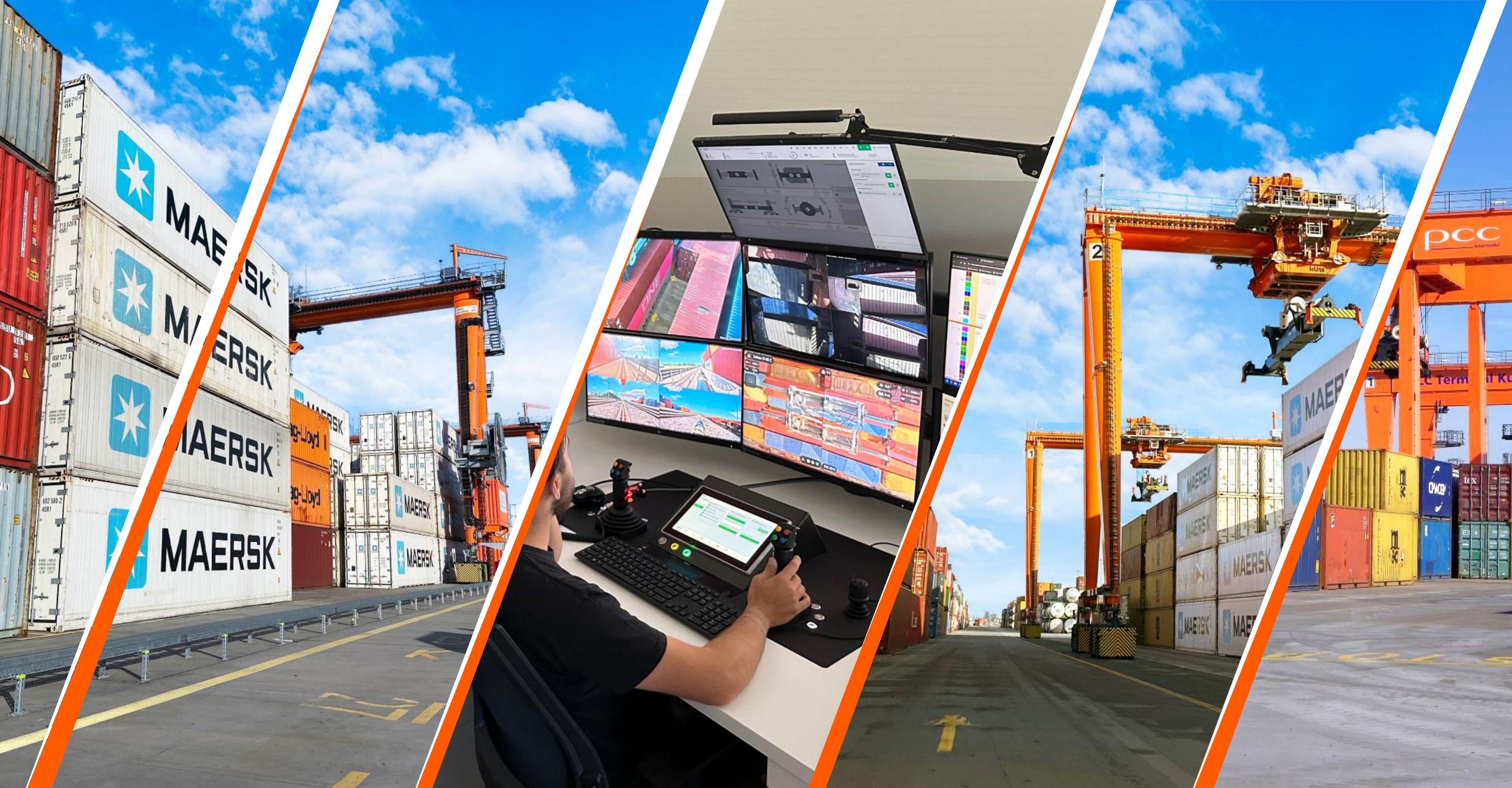
PCC Kutno Terminal
